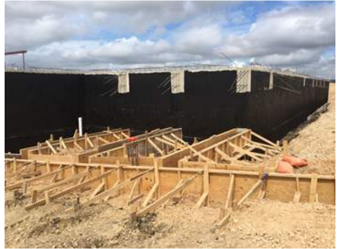
BUILDING TRANSITION BETWEEN LOWER AND UPPER LEVEL
