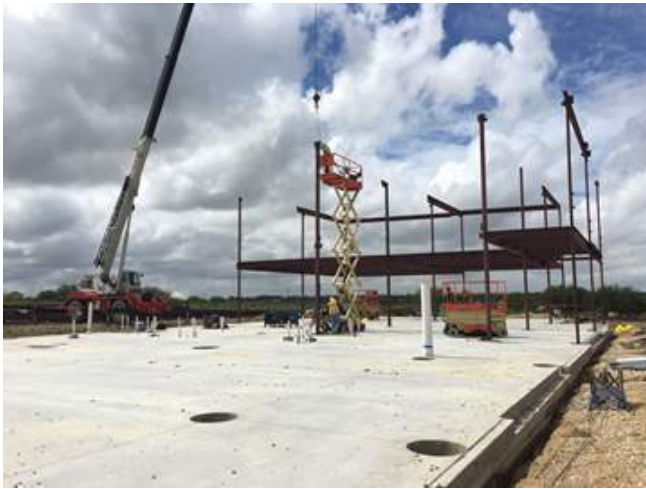
STRUCTURAL STEEL ERECTION UNDERWAY AT THE 2-STORY CLASSROOM WING
