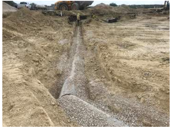
SITE UTILITIES, INCLUDING STORM SEWER INLETS AND PIPING IN PROGRESS
