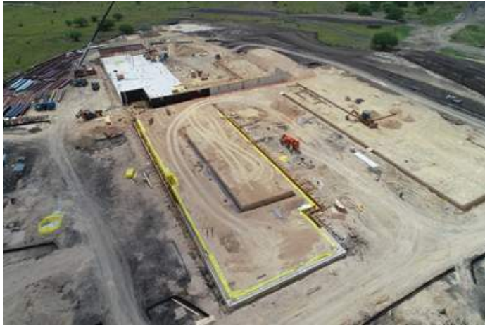
OVERALL VIEW OF THE BUILDING LOOKING SOUTH
